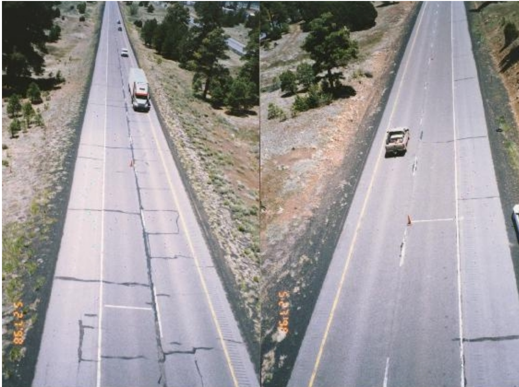
Figure 3 US Interstate 40 near Flagstaff, Arizona. 4” conventional asphalt (left) and 2” asphalt rubber overlays on Portland Concrete Cement placed in 1990, photo taken 1998.
