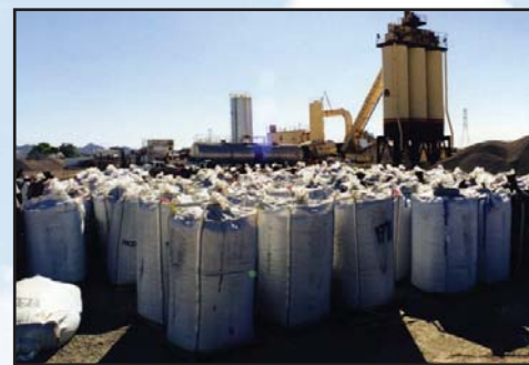
Rubber does not cause smoke at hot-plants. Above, a hot plant during production of A-R near Tucson, AZ.
