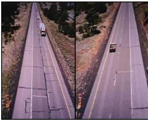
Conventional AC and A-R test sections placed on I-40 Flagstaff, AZ, 1990.
