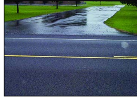
A dense graded surface is seen in the background during a light rain, the rubber is in the foreground, photo courtesy of Tenn. DOT.
