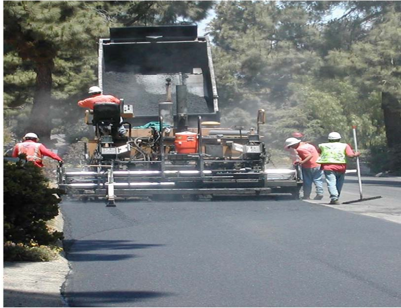
Figure 5. Typical asphalt rubber mix paving.
