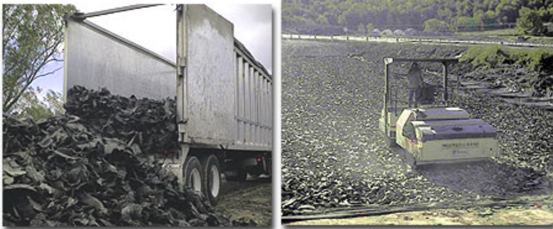
Figure 3. Tire shreds for alternate daily cover. Tire shreds being placed as cover or fill.
